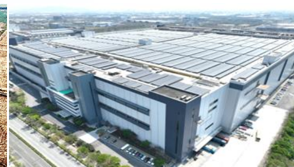
群創光電 23,800kWp
